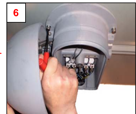
Secure guard using the 5mm Allen Key 'T' Bar supplied.
